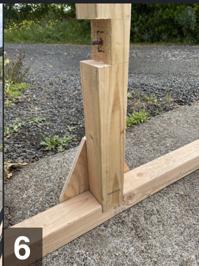
6 Bolts Connections connect posts to beams.
