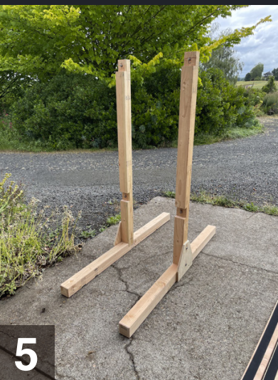
5 Knotched Posts accept beams (lap joints).
