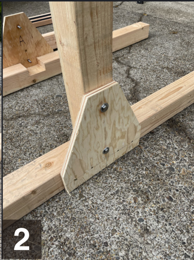
2 Plywood Braces are screwed to bases.
